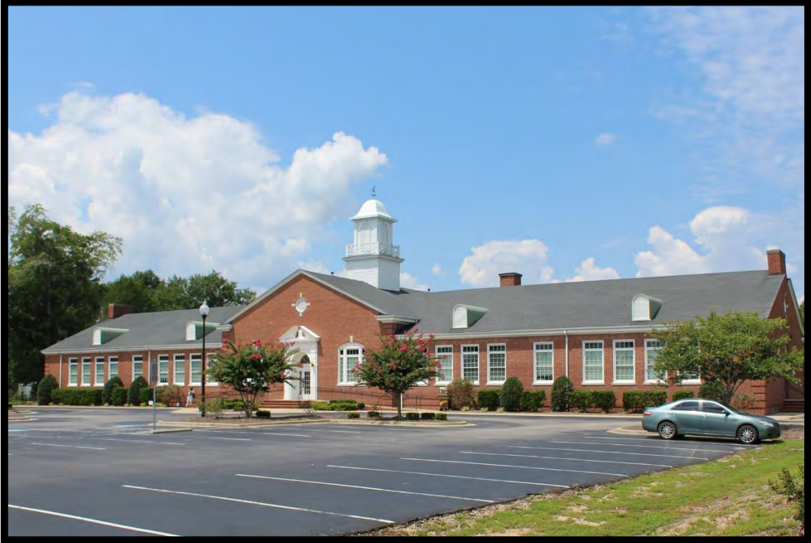
Figure 57: Eastover Elementary School (CD0164).
