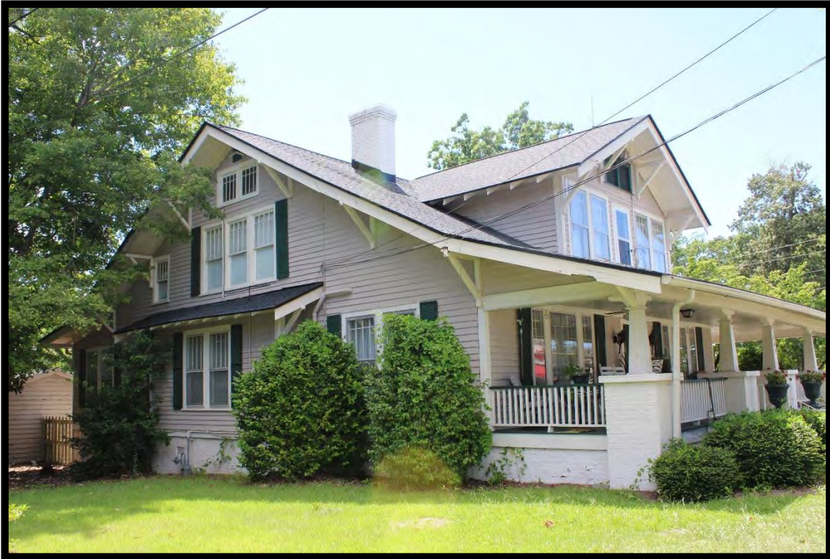
Figure 122: W. P. Lee House, Looking West.
