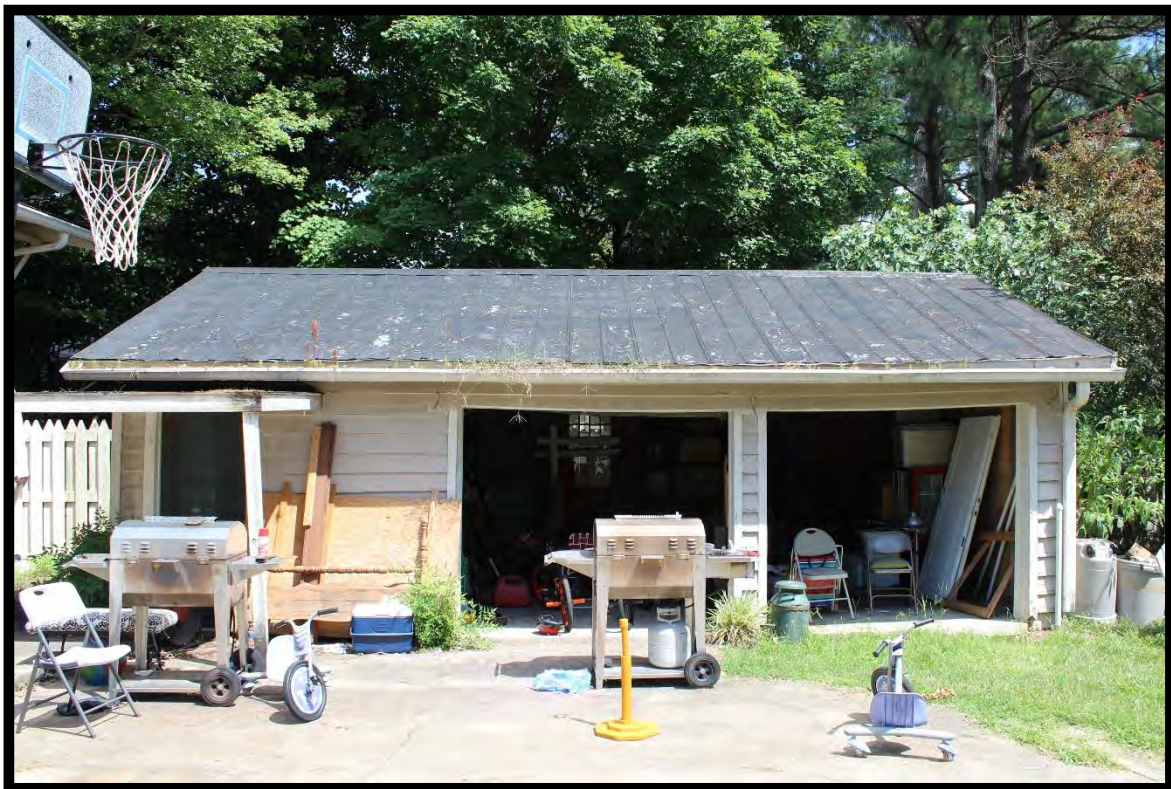
Figure 123: W. P. Lee House, Looking Southeast.
