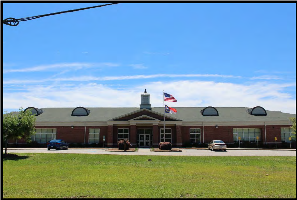
Figure 41: New Eastover-Central Elementary School Building, Looking Southeast.
