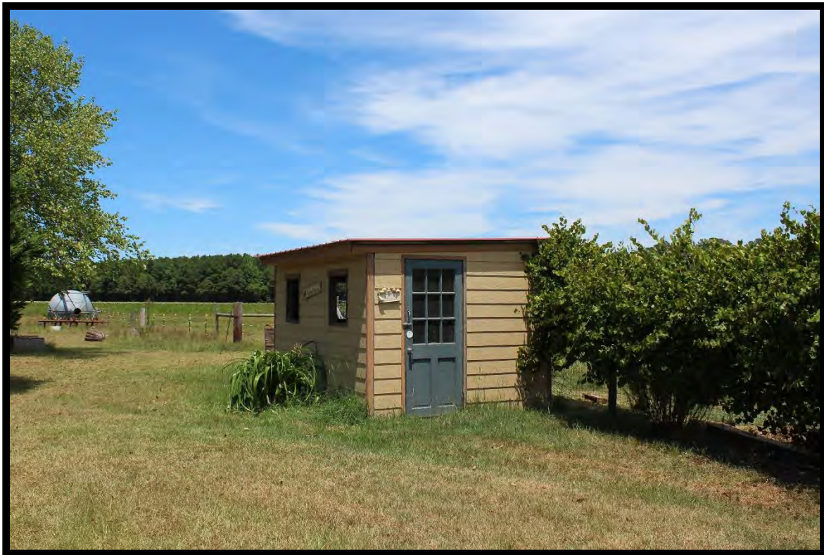
Figure 88: Chicken House, Honeycutt House, Looking Northeast.
