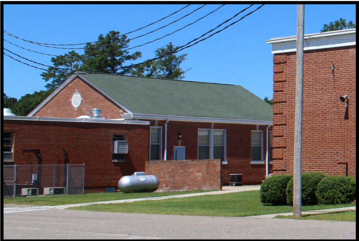
Figure 24: Cafeteria, Central High School, Looking East.
