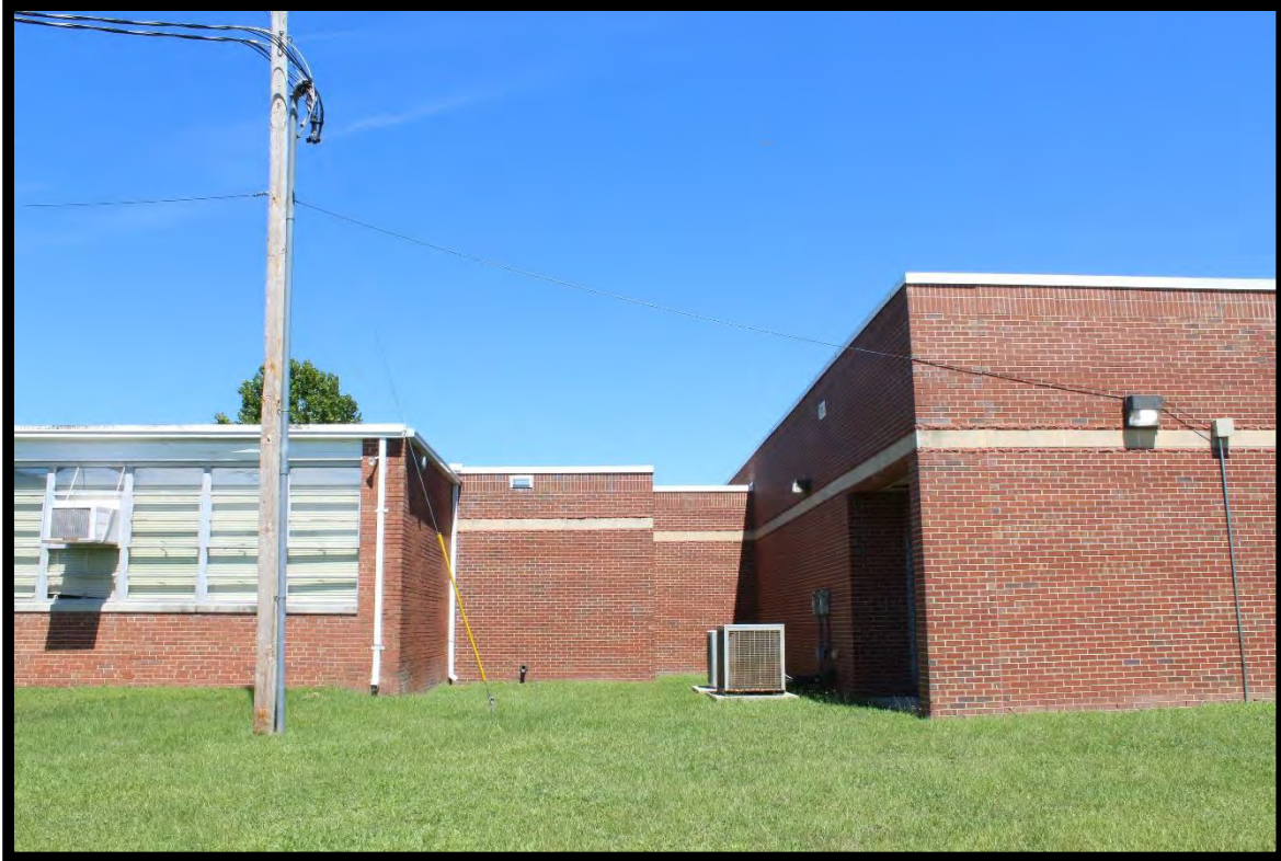
Figure 37: Library Addition, Central High School, Looking Northwest.
