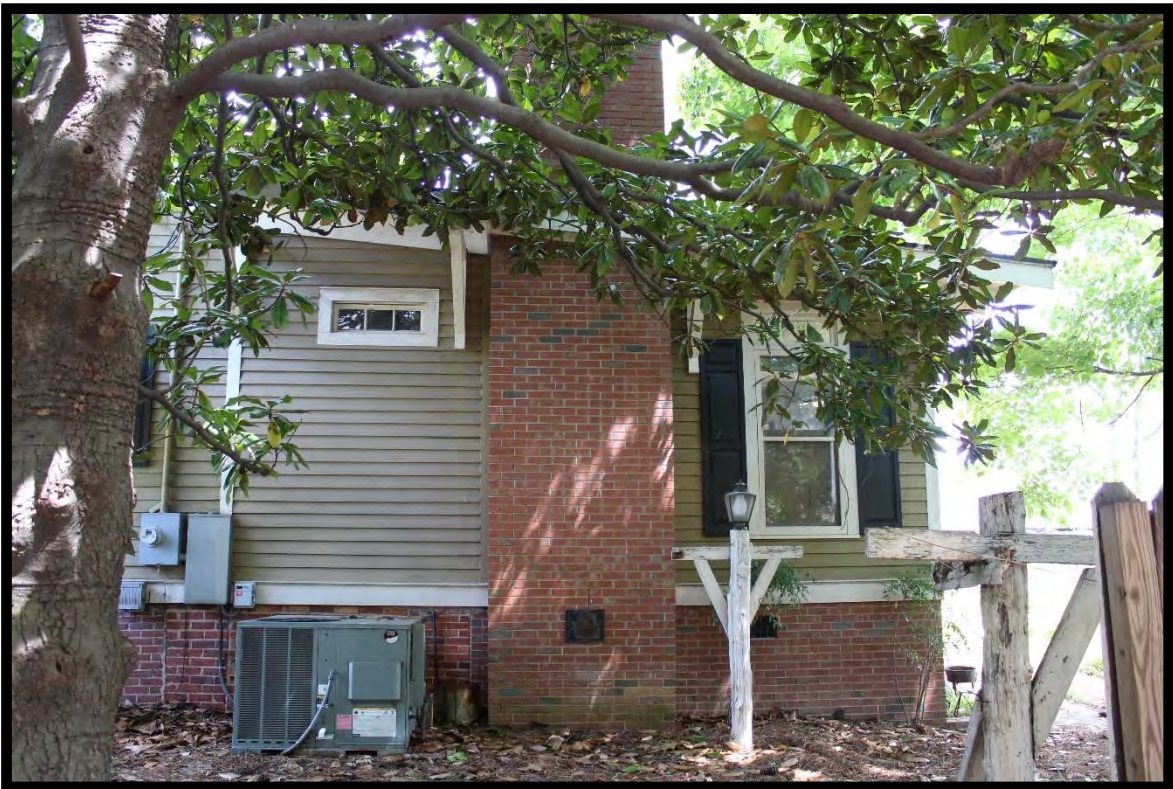
Figure 98: Uriah James Tart House, Looking Southeast.
