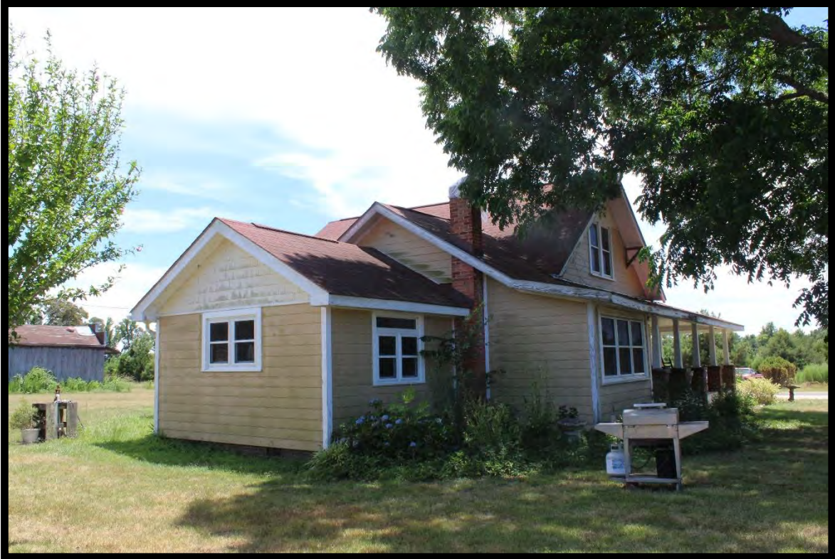
Figure 82: Honeycutt House, Looking South.
