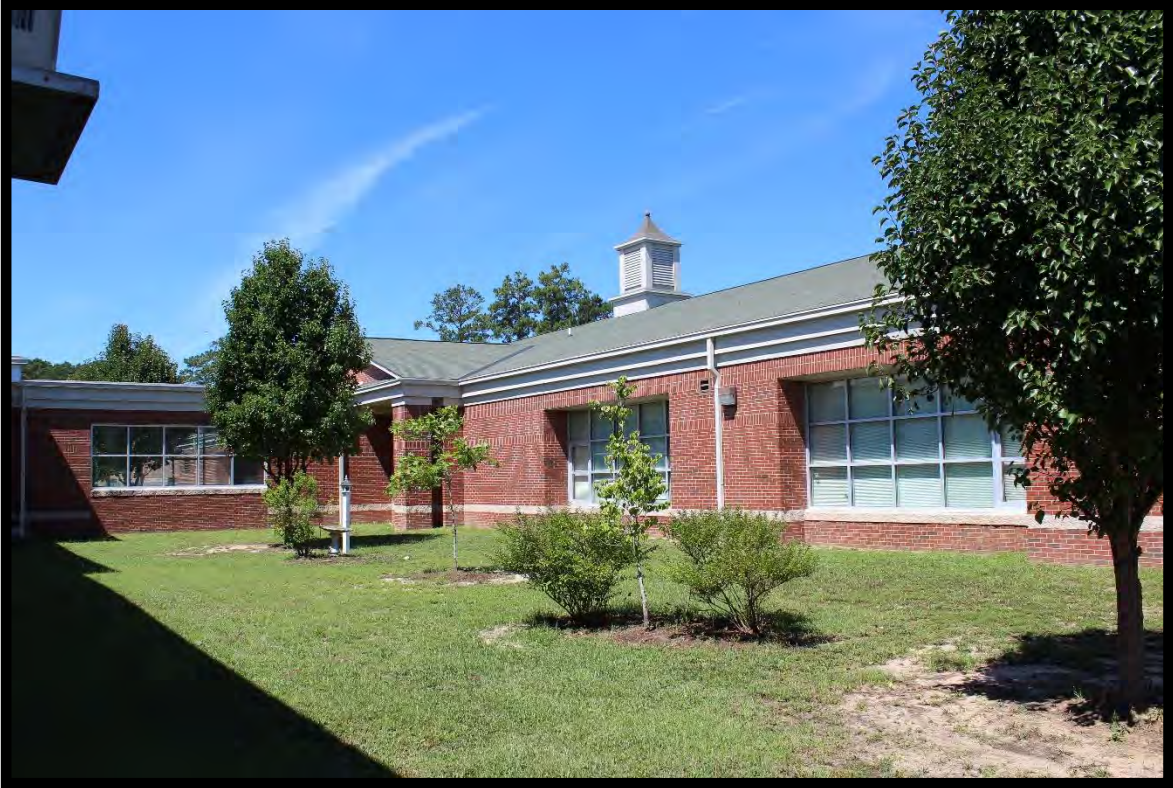
Figure 43: New Eastover-Central Elementary School Building, Looking Northwest.
