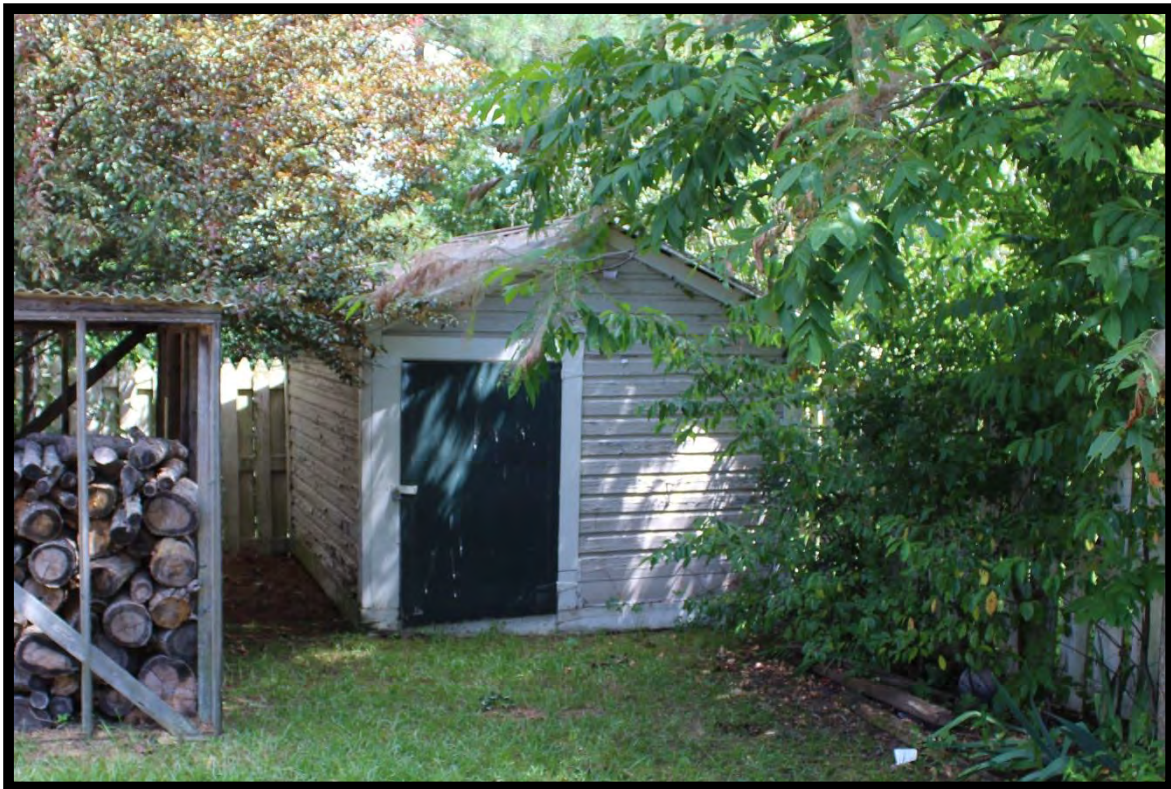
Figure 125: Uriah James Tart House, Looking Southeast.
