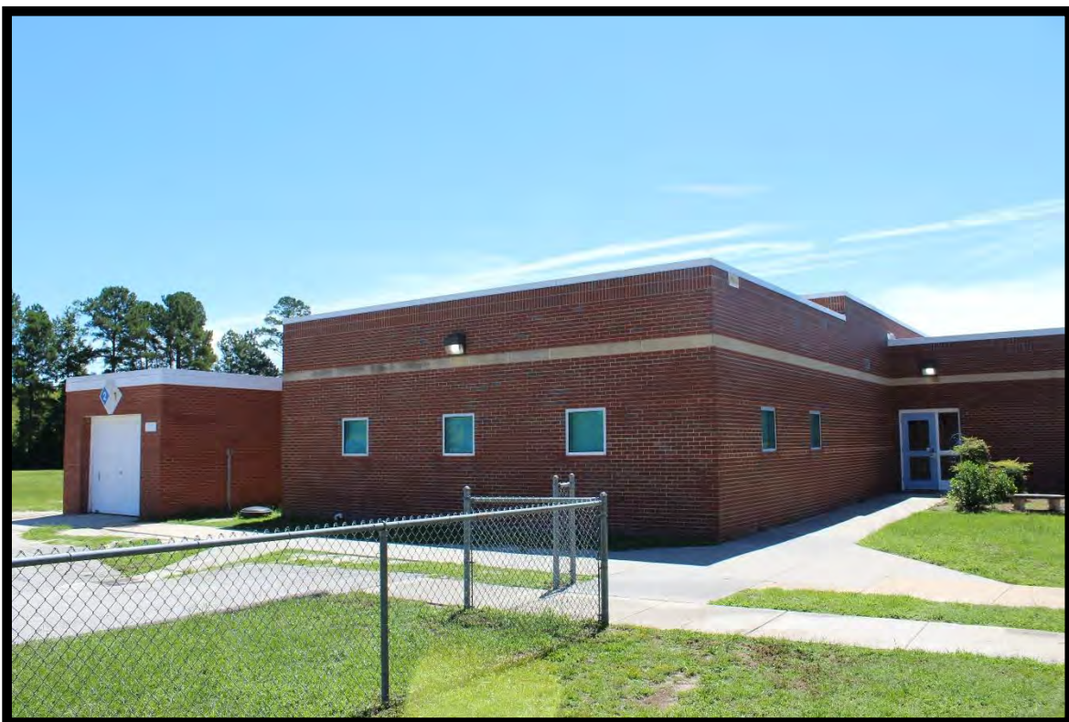
Figure 34: Library Addition, Central High School, Looking East.
