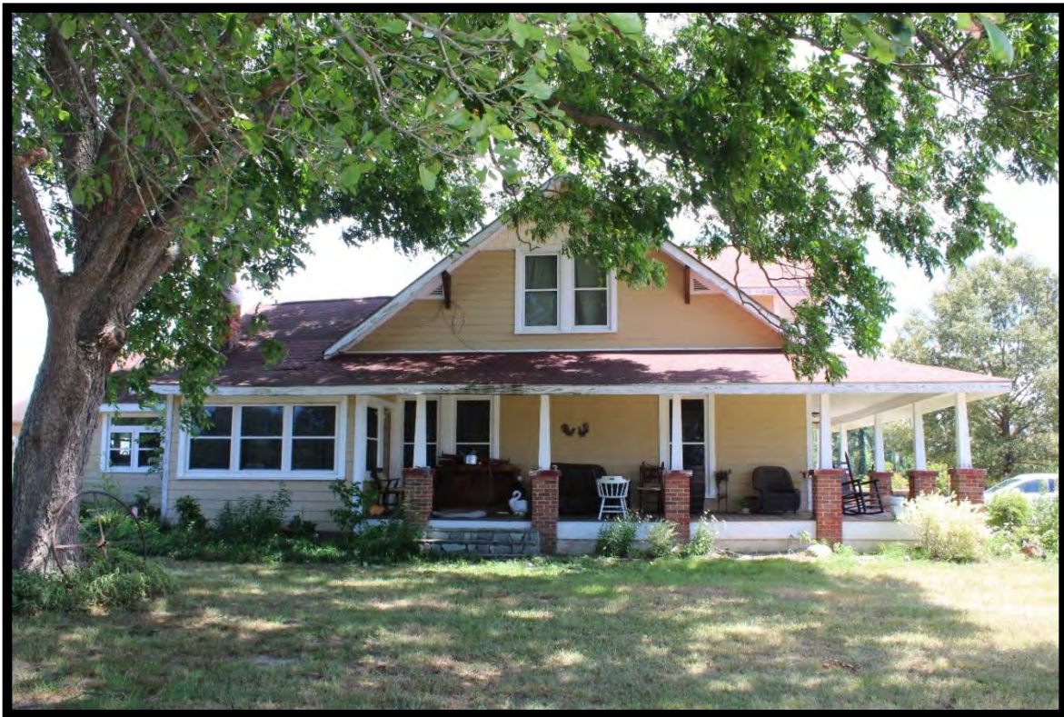
Figure 81: Honeycutt House, Looking Southeast.
