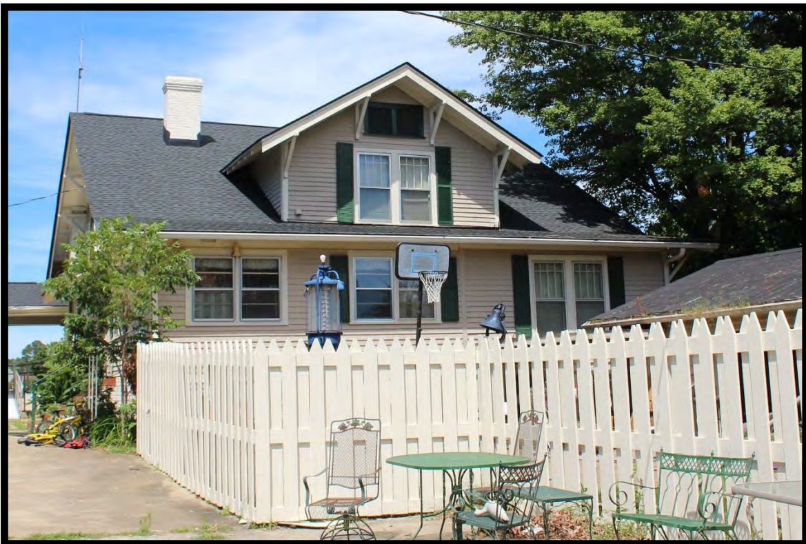
Figure 121: W. P. Lee House, Looking Northeast.
