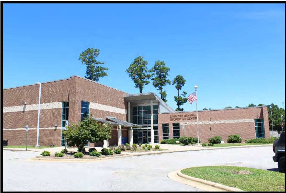
Figure 45: Eastover Recreational Center, Looking Northwest.
