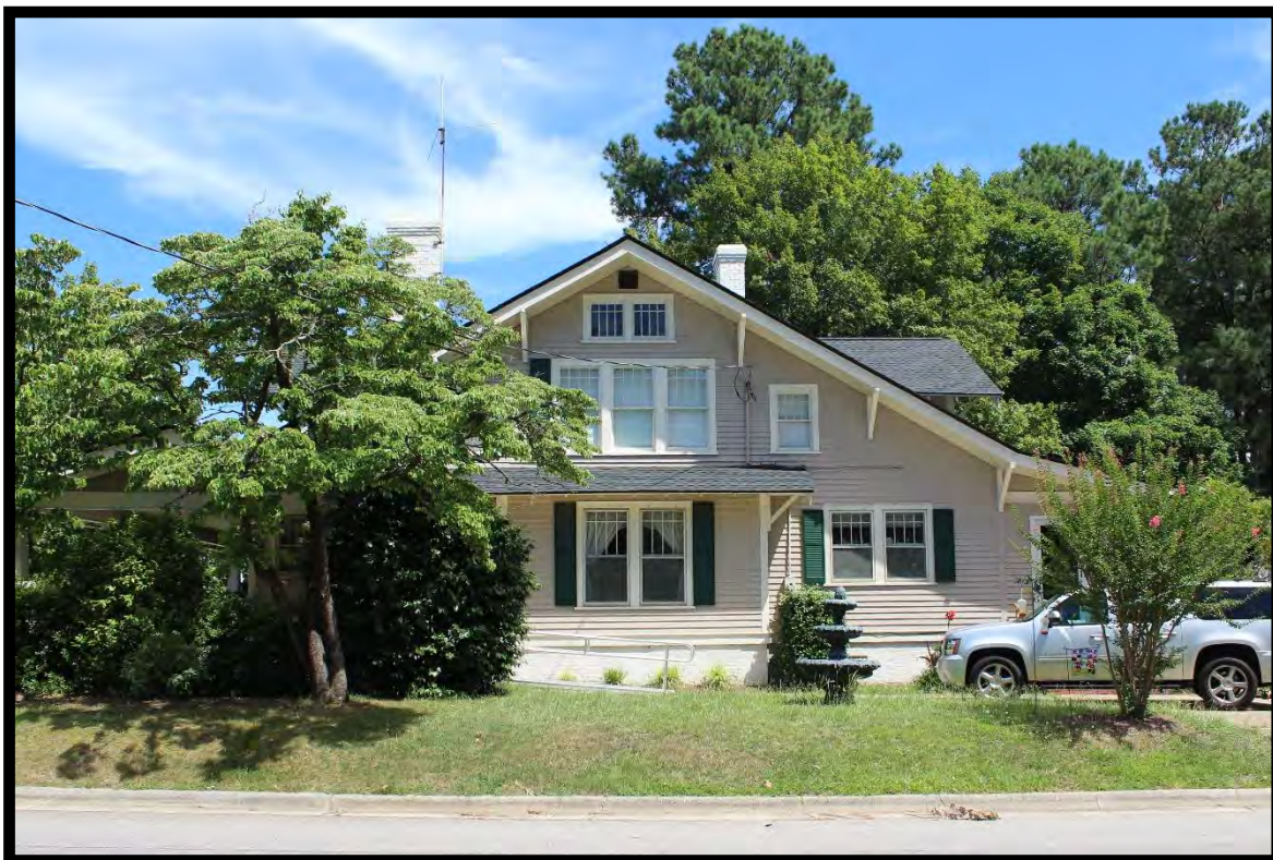
Figure 119: W. P. Lee House, Looking Southeast.
