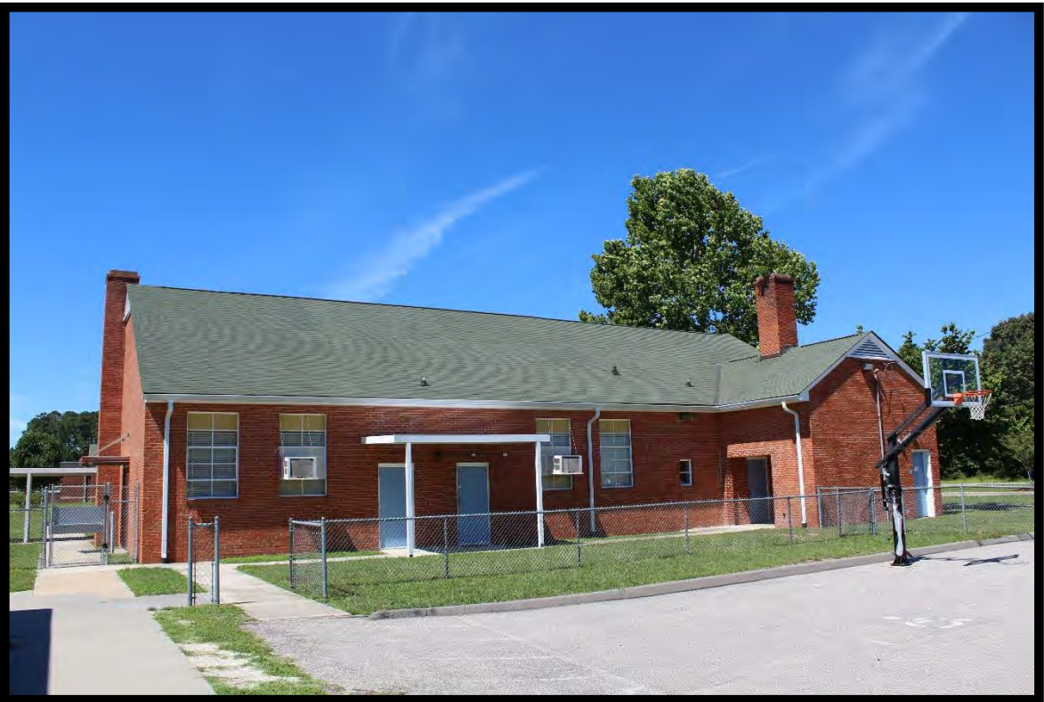
Figure 8: Agricultural Building, Central High School, Looking West.
