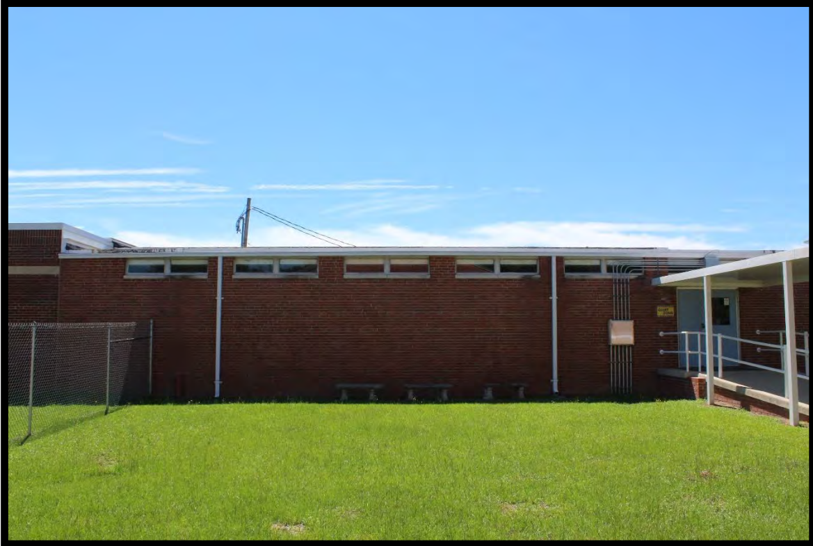
Figure 32: Northeast Addition, Central High School, Looking Southeast.
