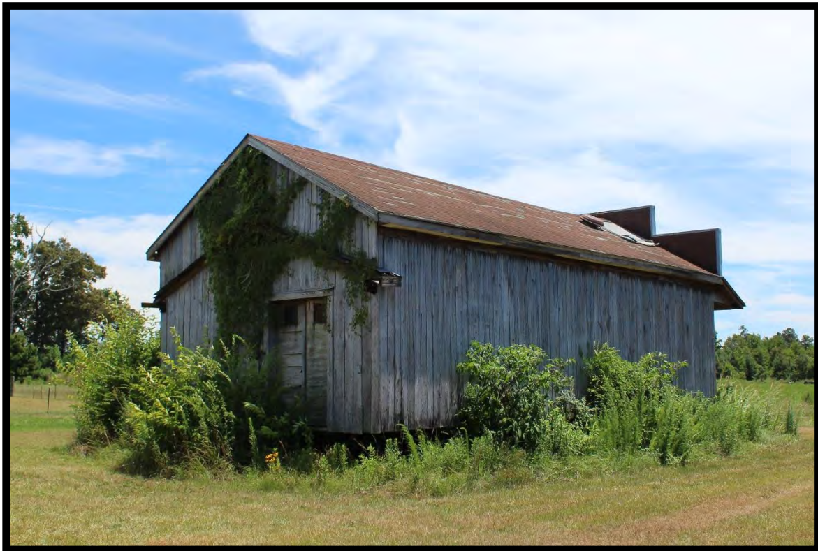
Figure 86: Store, Honeycutt House, Looking South.
