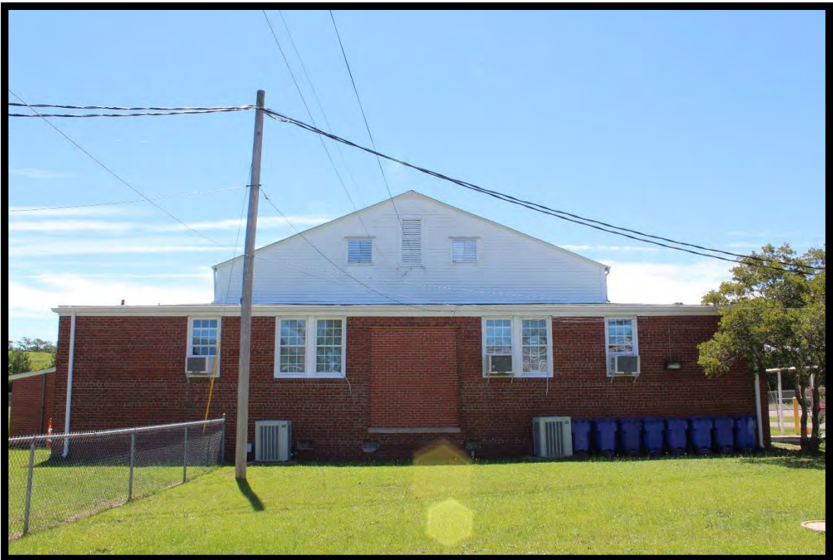
Figure 16: Gymnatorium, Central High School, Looking Southeast.
