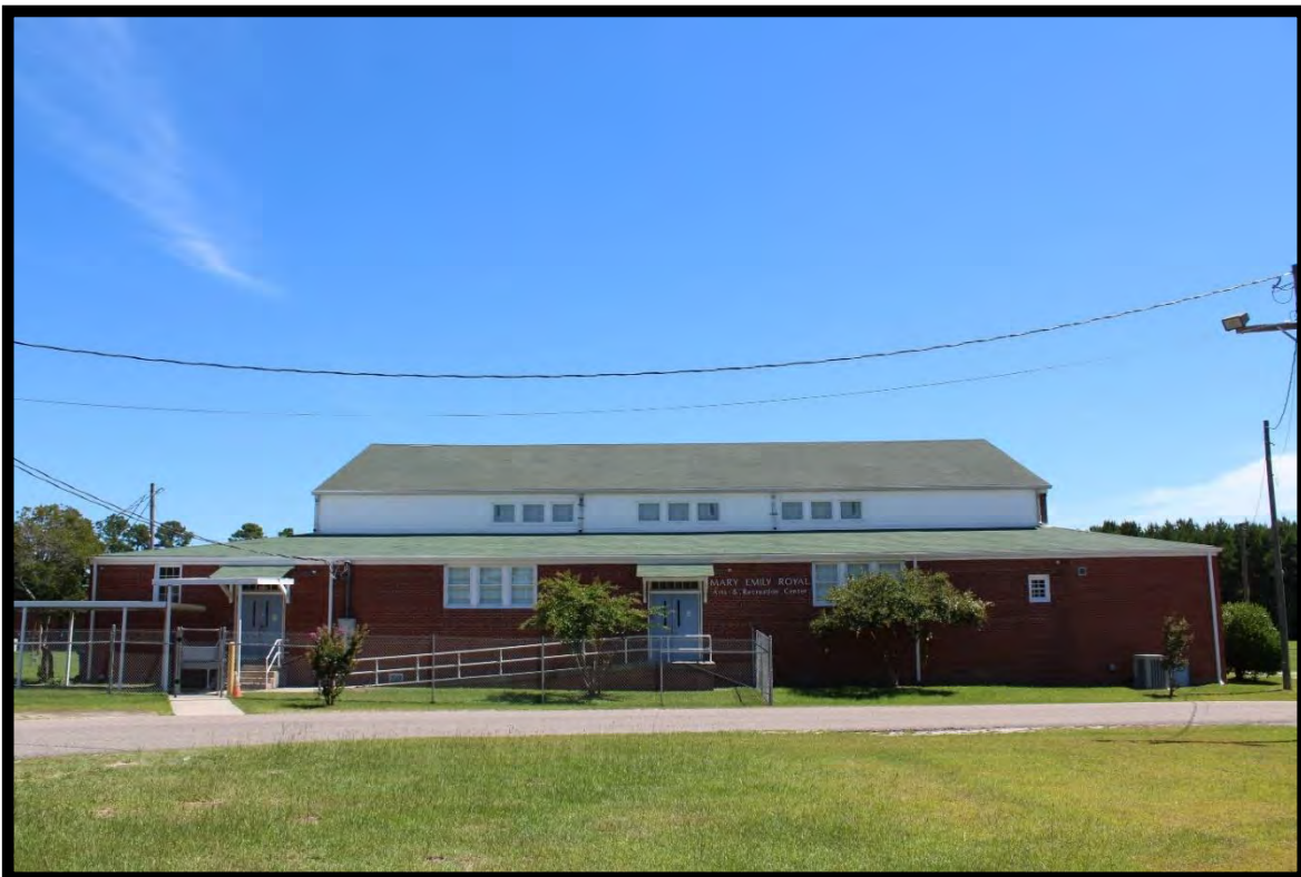
Figure 13: Gymnatorium, Central High School, Looking Northeast.
