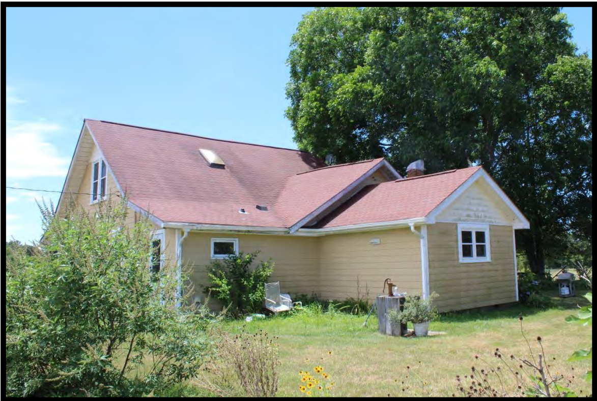
Figure 83: Honeycutt House, Looking Southwest.
