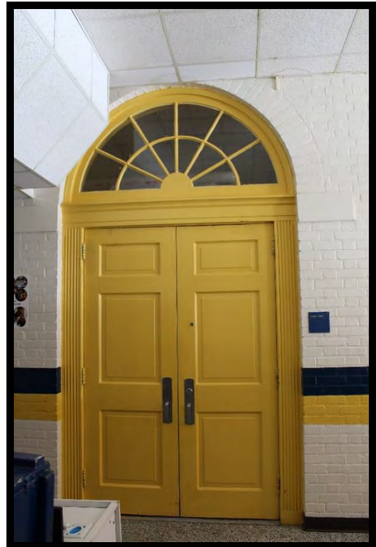
Figure 22: Cafeteria, Looking Southeast.
