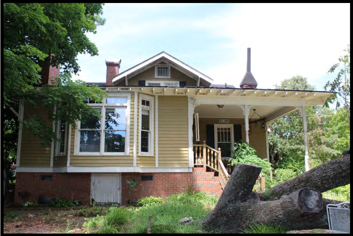
Figure 99: Uriah James Tart House, Looking Northeast.
