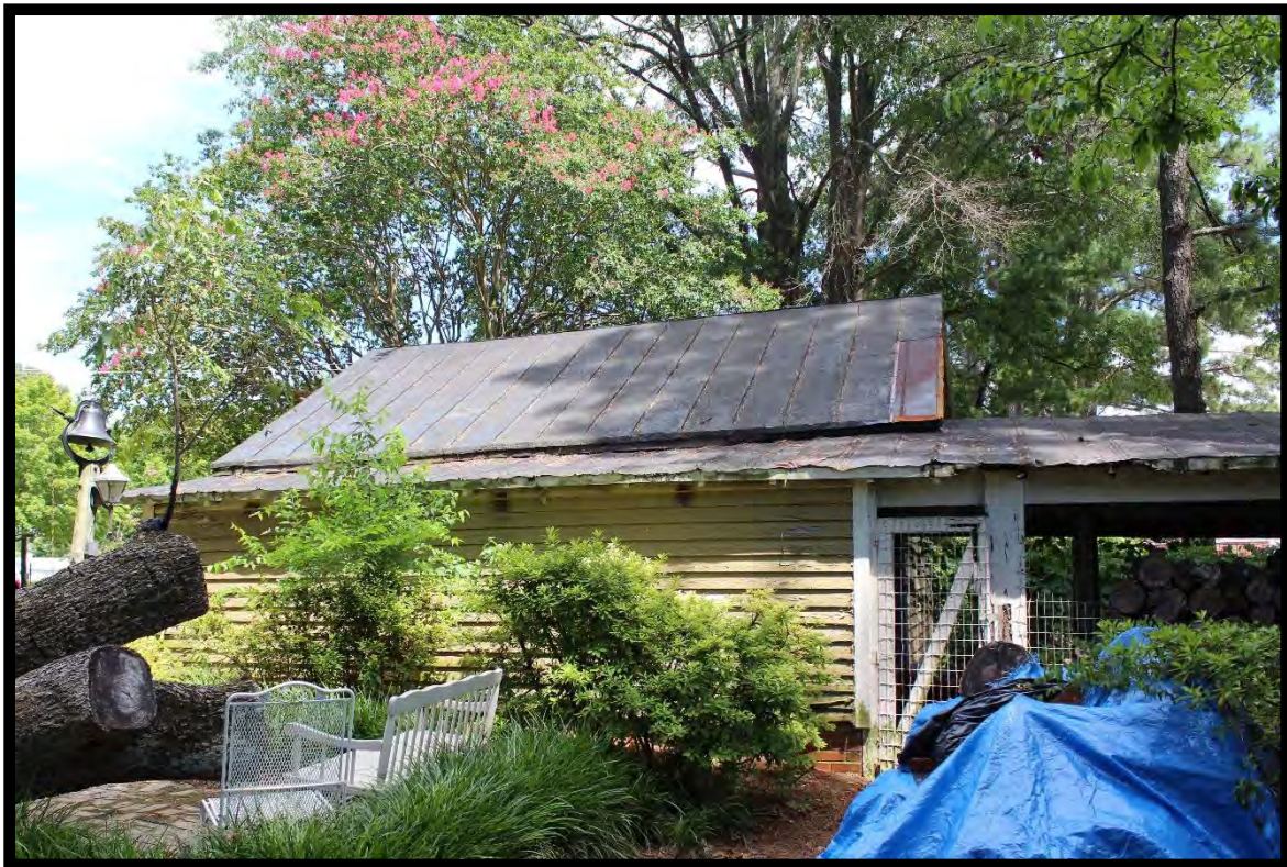
Figure 103: Garage, Uriah James Tart House, Looking Southeast.
