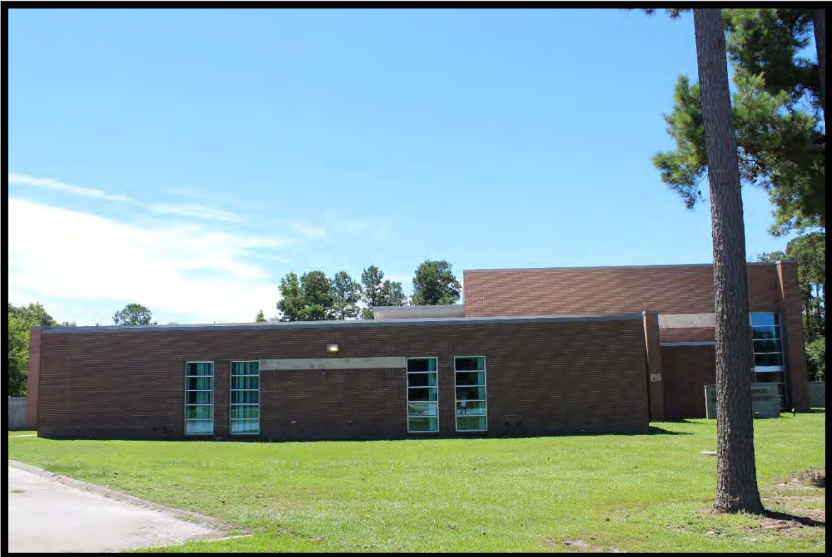
Figure 47: Eastover Recreational Center, Looking South.
