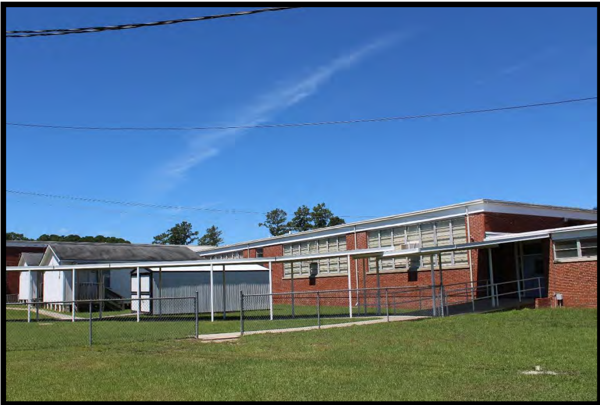
Figure 29: Classroom Wing, Central High School, Looking Southwest.
