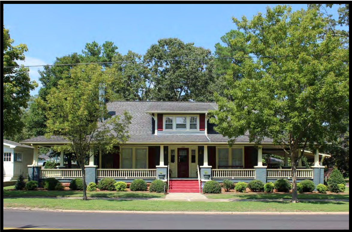
Figure 130: Farmer House, 300 West Main Street, Benson, NC (JT0507).
