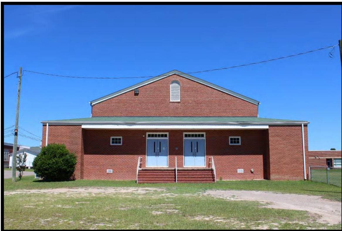
Figure 14: Gymnasium, Central High School, Looking Northwest.
