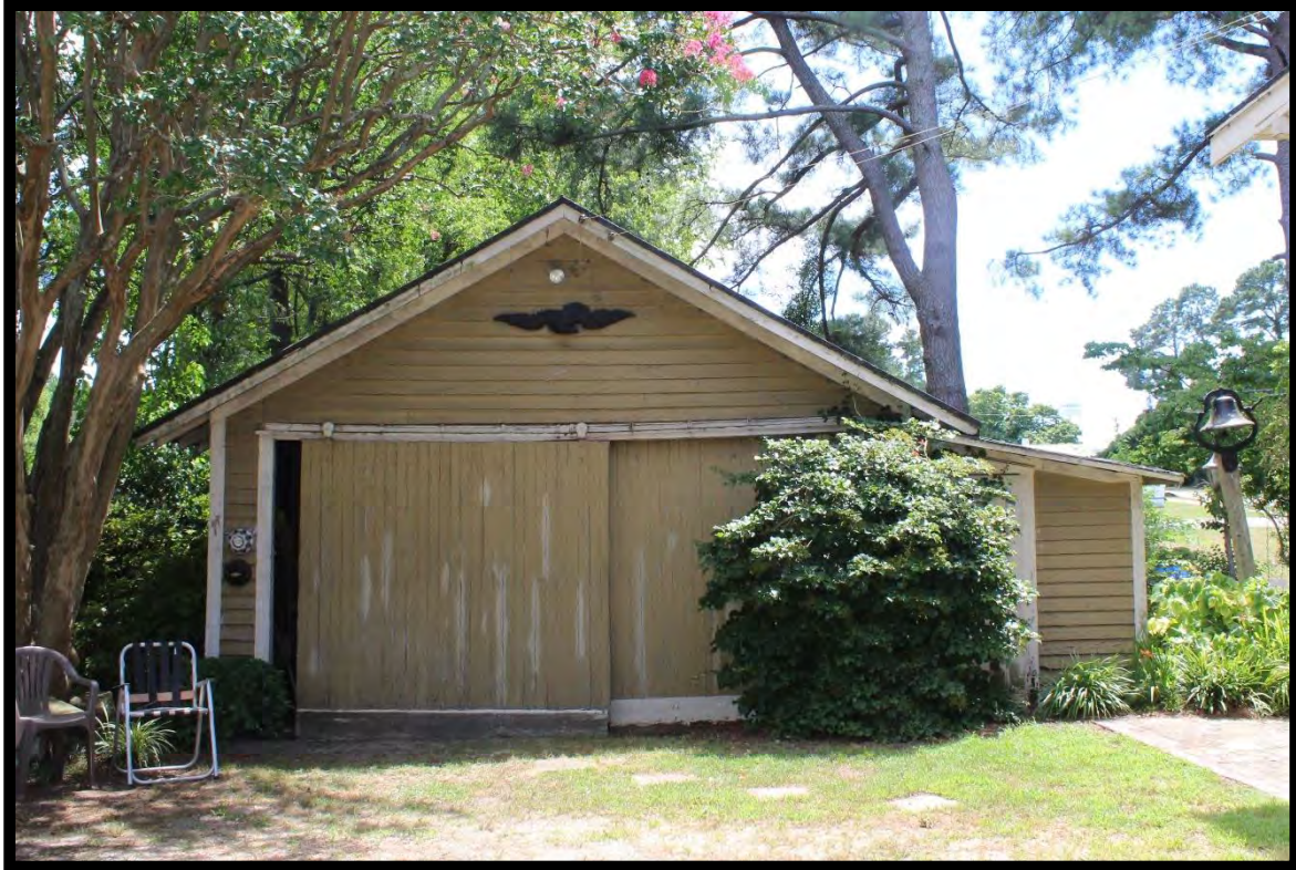
Figure 102: Garage, Uriah James Tart House, Looking Southwest.
