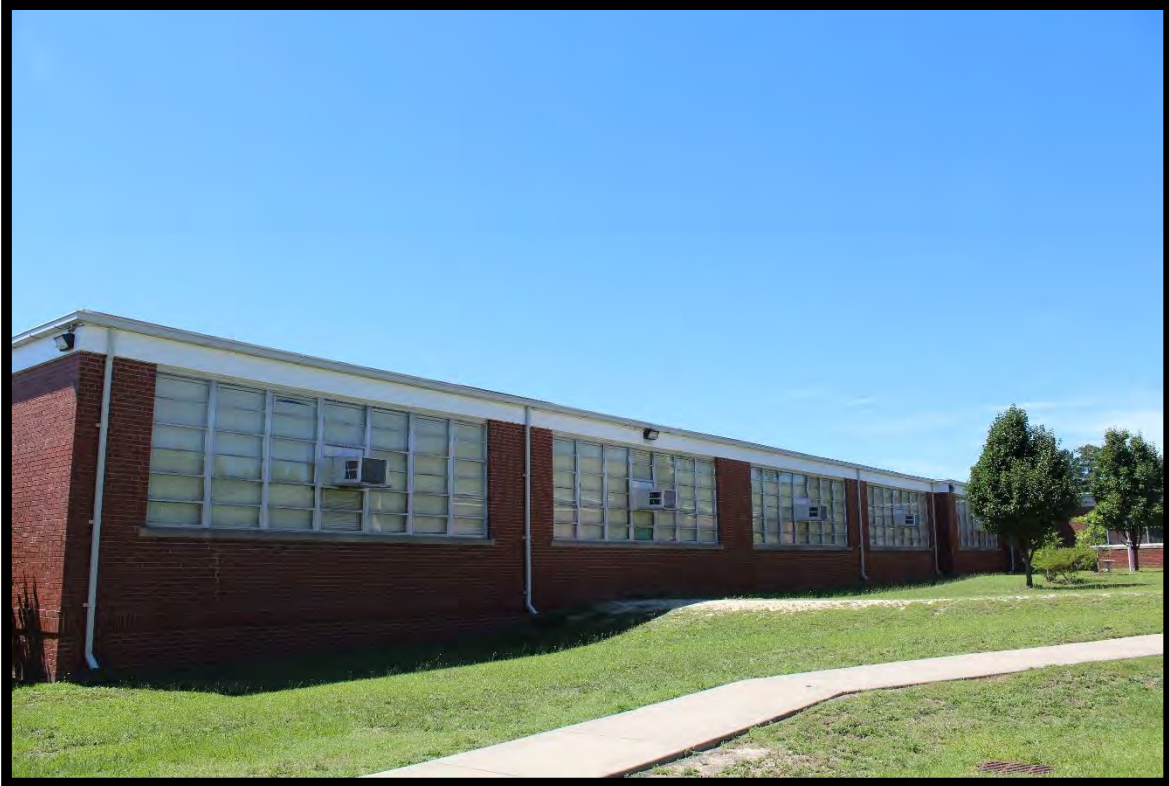
Figure 28: Classroom Wing, Central High School, Looking South.
