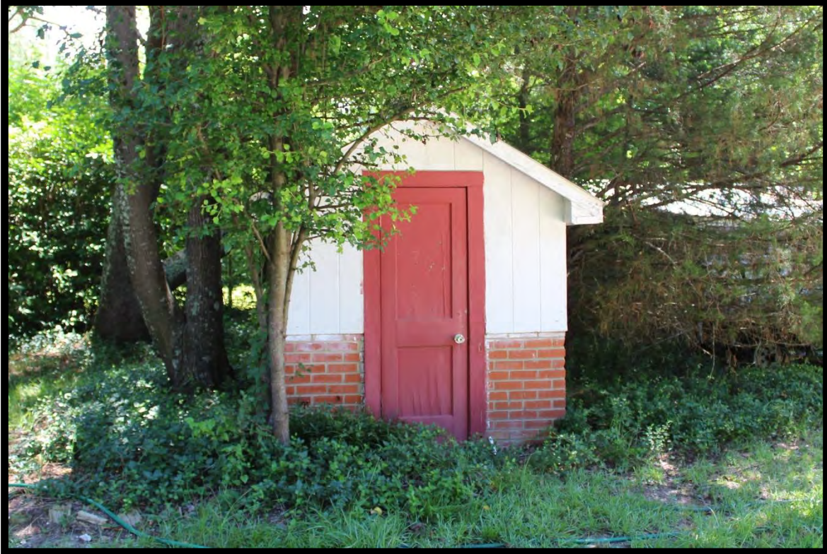
Figure 66: Wellhouse, Blue-Collier House, Looking South.
