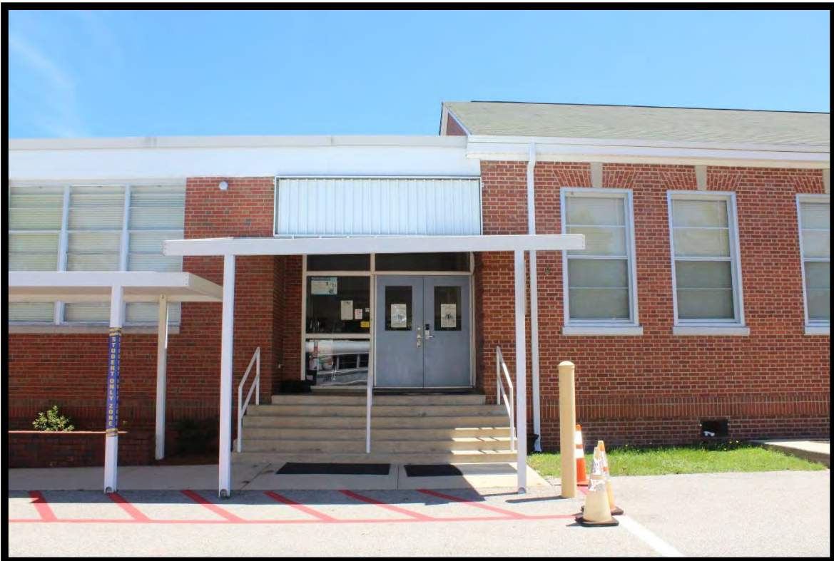
Figure 39: Southwest Addition, Central High School, Looking Northeast.
