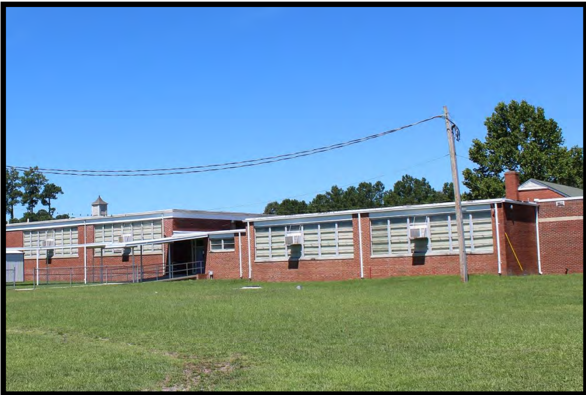
Figure 33: Northeast Addition, Central High School, Looking West.
