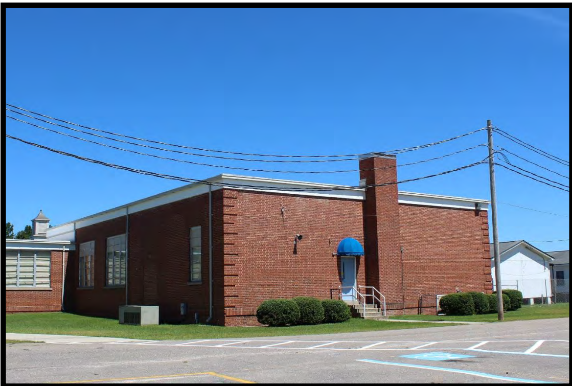
Figure 31: Kindergarten Wing, Central High School, Looking North.
