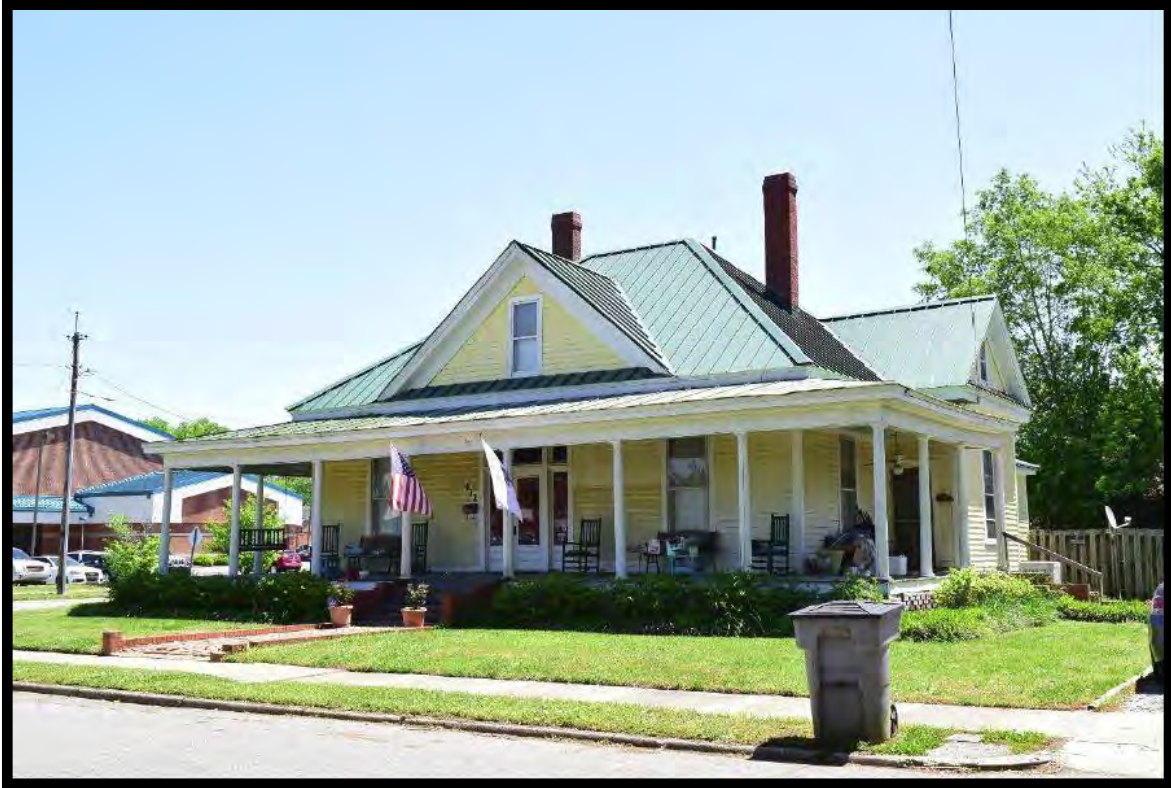
Figure 77: 412 N. Massey Street, Selma, NC (JT0088).
