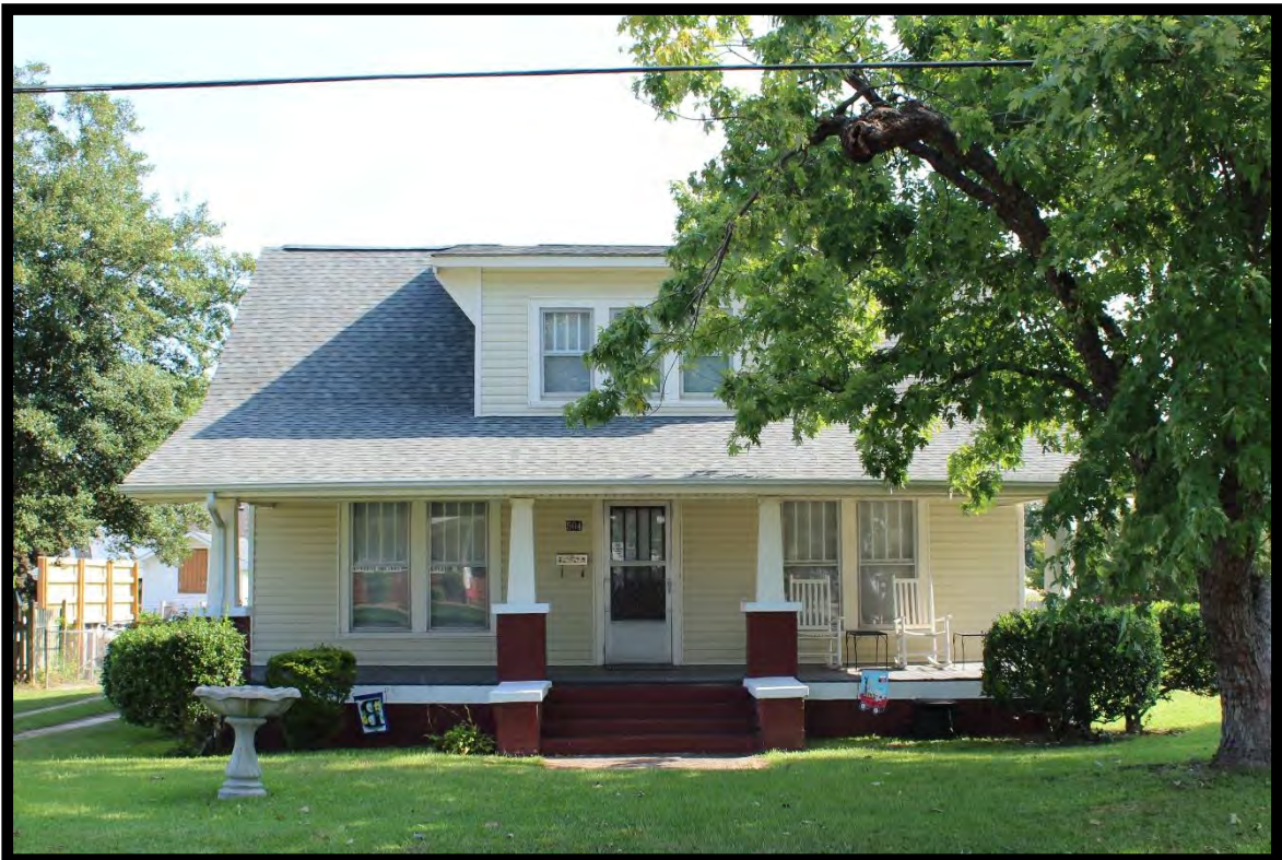
Figure 115: 504 West Parrish Drive, Benson, NC (JT0600).
