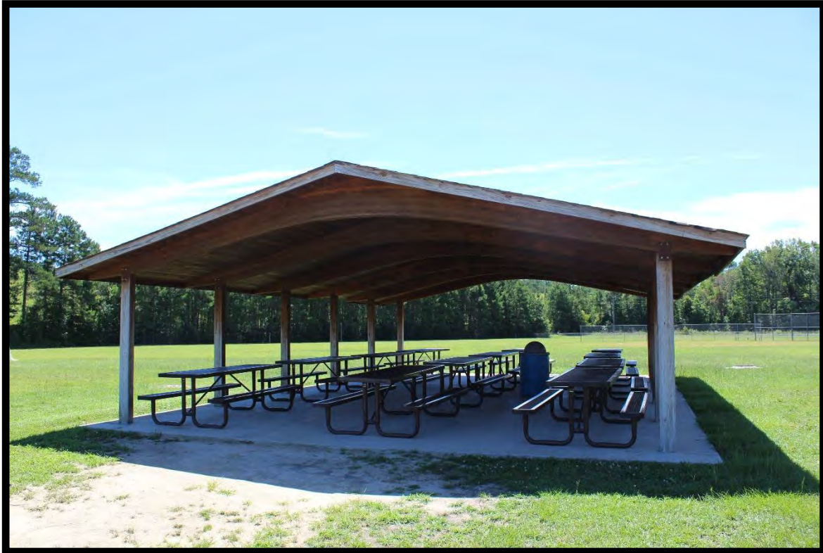
Figure 49: Picnic Shelter, Central High School, Looking East.
