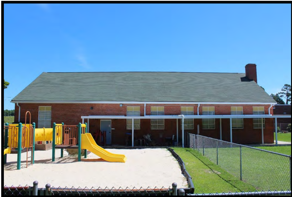
Figure 10: Agricultural Building, Central High School, Looking Northeast.
