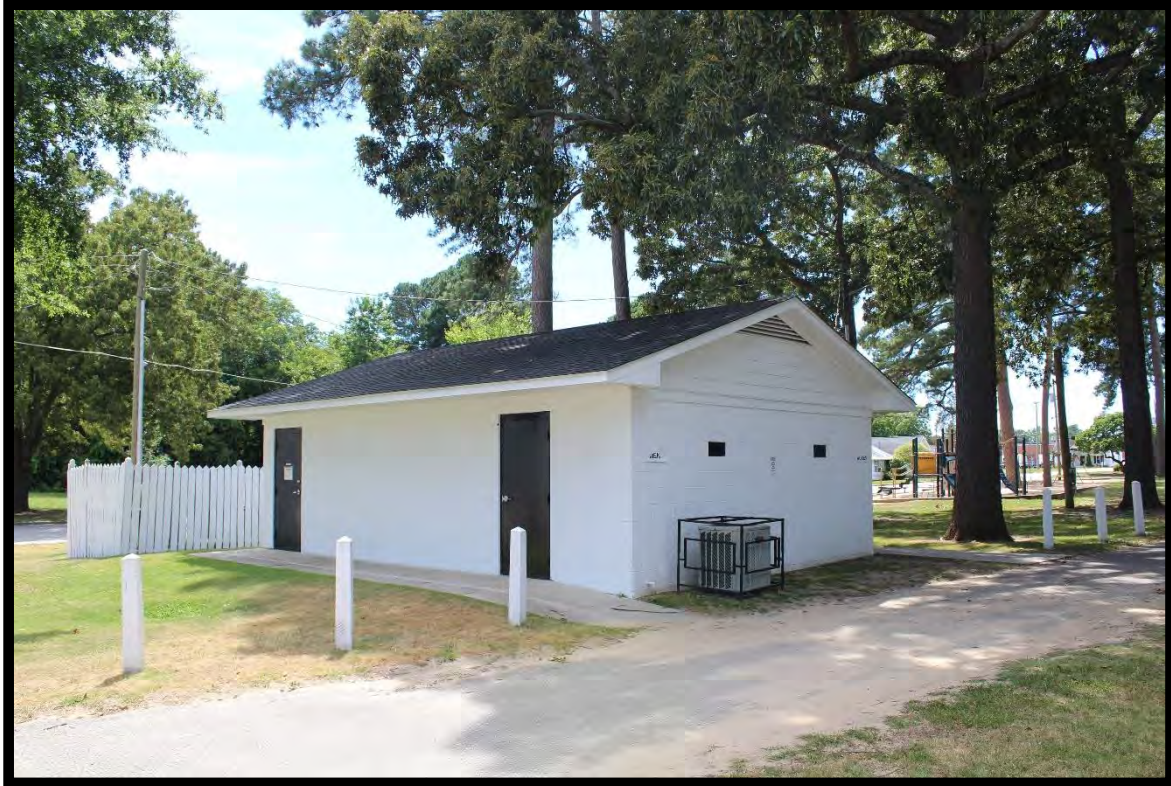
Figure 140: Restrooms, Benson Singing Grove, Looking East.
