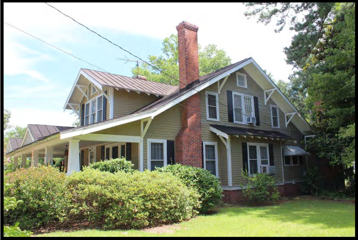
Figure 97: Uriah James Tart House, Looking South.
