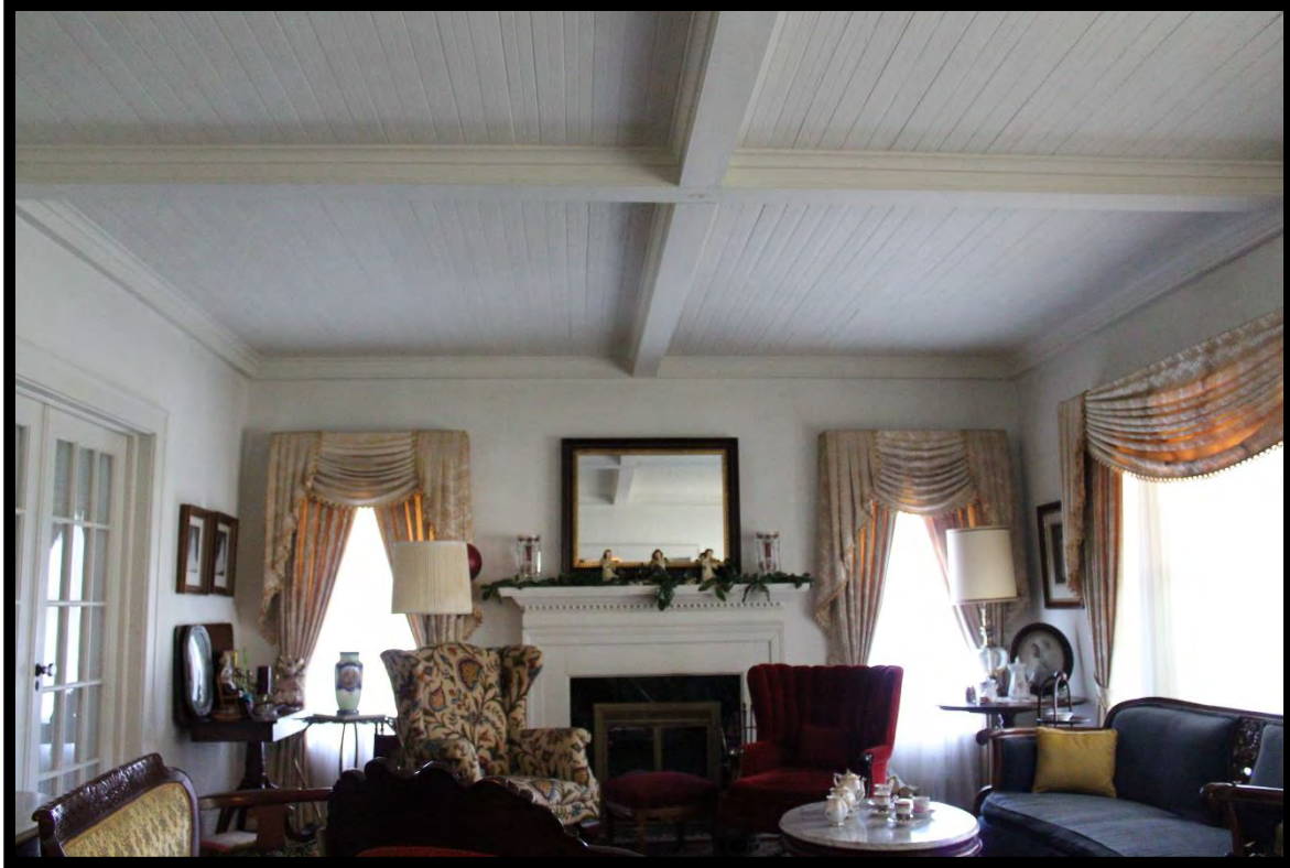
Figure 106: Beaded Ceiling with Exposed Beams, Uriah James Tart House.
