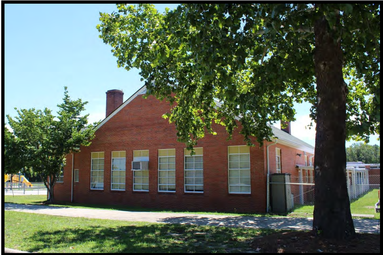
Figure 5: Agricultural Building, Central High School, Looking East.
