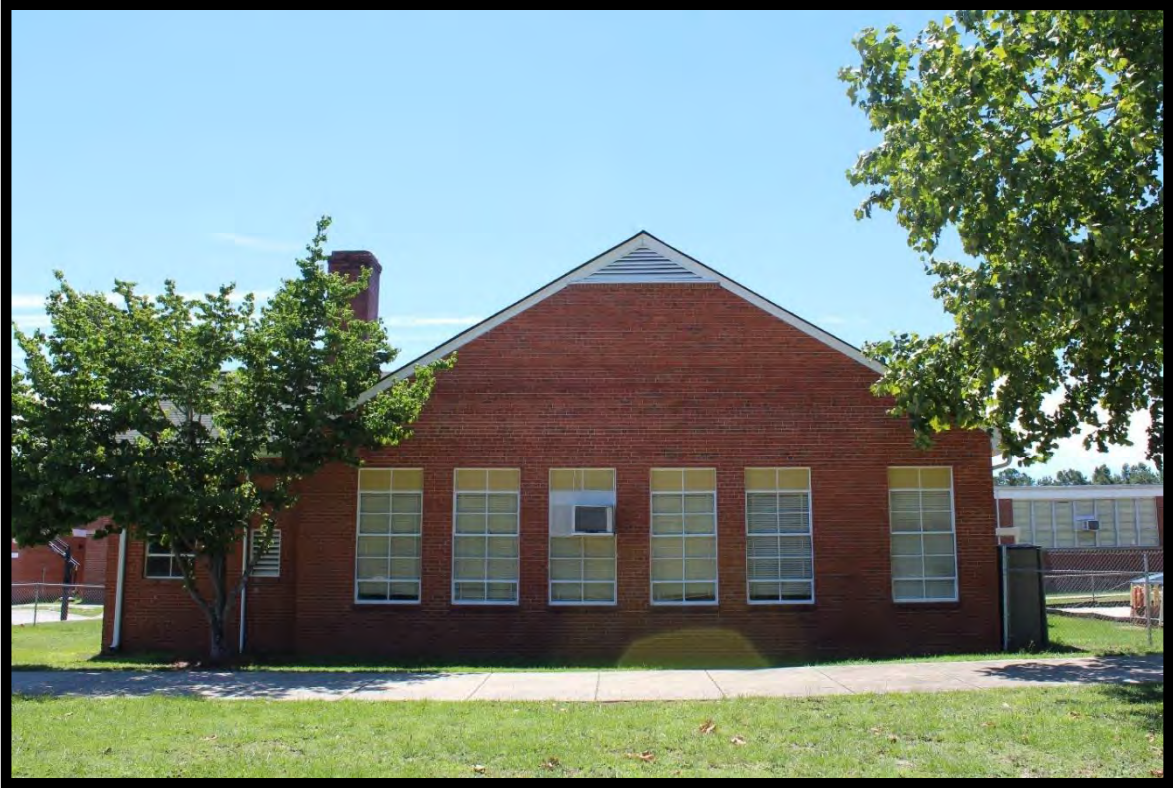
Figure 7: Agricultural Building, Central High School, Looking Southeast.
