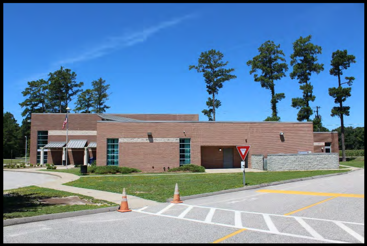
Figure 48: Eastover Recreational Center, Looking West.
