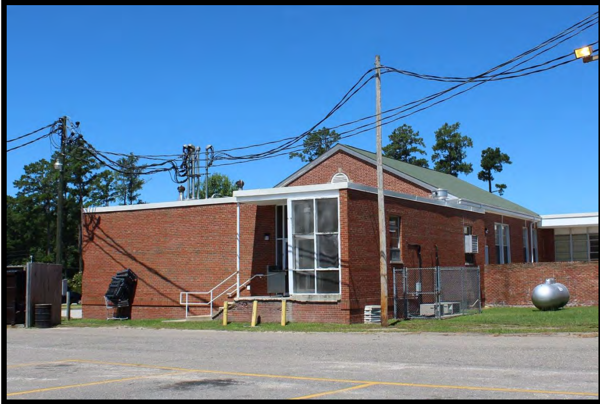
Figure 25: Cafeteria/Kitchen Addition, Central High School, Looking East.
