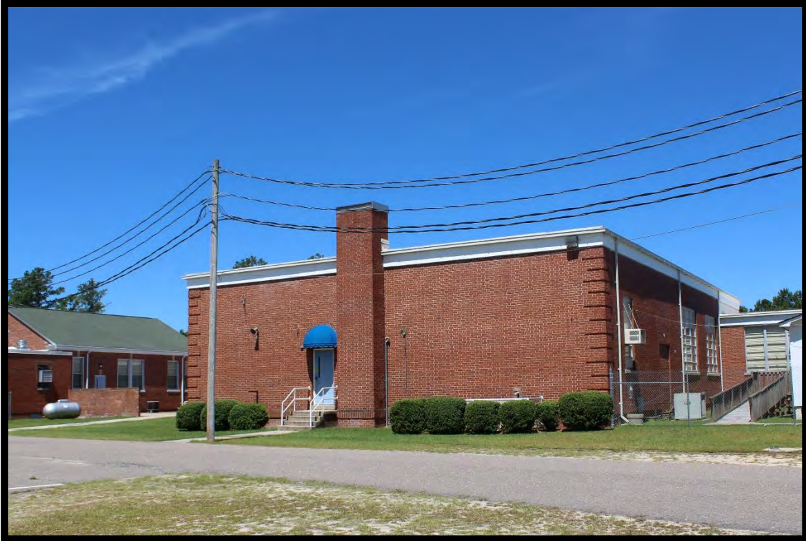
Figure 30: Kindergarten Wing, Central High School, Looking West.
